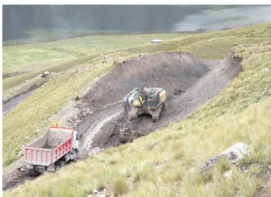
a. Slope profiling
