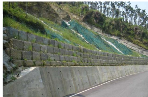
b. Gabion systems
