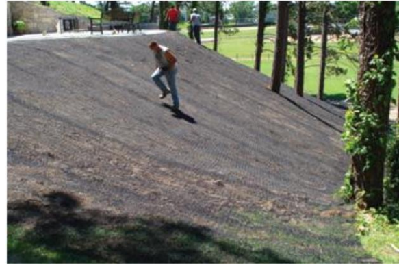
d. Reinforcement mat
